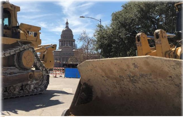
Picture from the Capitol Complex construction project.
