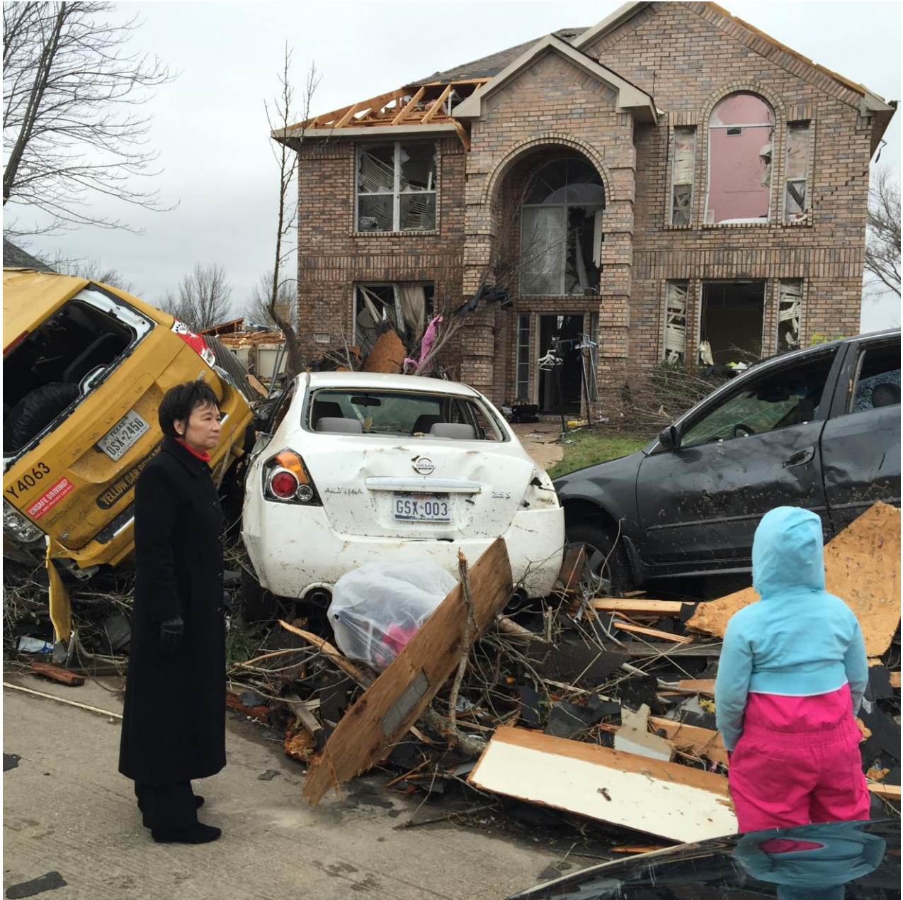
Surveying the Damage from the December 26th Tornado in Garland.
